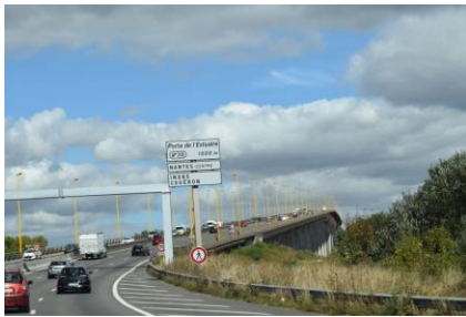
Broen i Nantes over Loire
