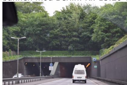
Tunnel under Tegel
